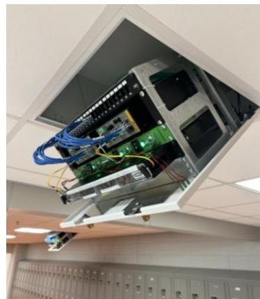
"With each singlemode fiber pair capable of supporting 100 Gigabits and each copper pair delivering 600 Watts, our Edge IDFs provide a total potential of 300 Gigabits of bandwidth and 1800 Watts of power—enough for the infrastructure to last at least 50 years," explains Hanshaw. "The switches also have unused ports and available PoE capacity, providing immediate means for us to connect new devices."
